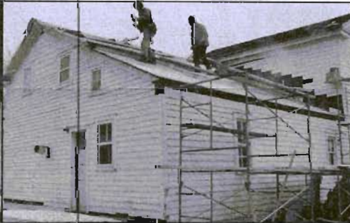
Roof sag repaired, new cedar shake roof installed.
