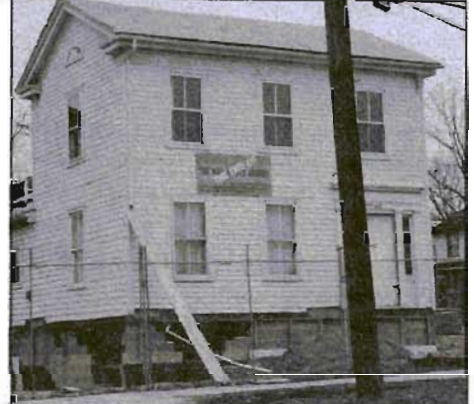
An abandoned gas station at Beakes and North Main Streets (top left) was cleared away by the City of Ann Arbor to make way for the WCHS Museum on Main Street. The house rode on steel beams (far left) to its new site.
