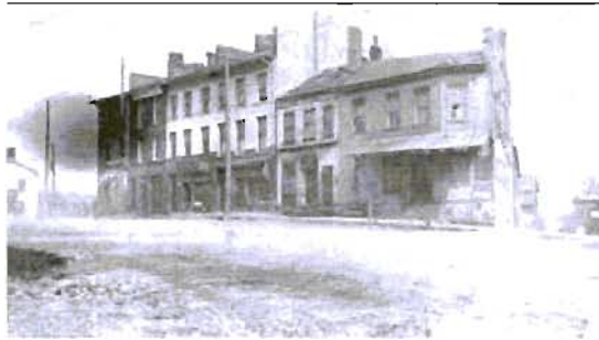
Huron Block, built by Josiah Beckley in Lower Town
