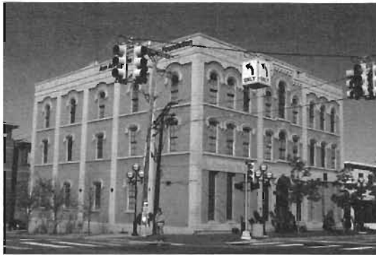
The Dobson McComber Building
