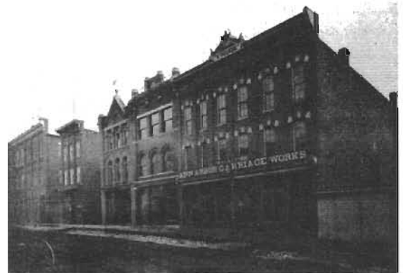
Harrier and Walker Buildings in the 1800s
